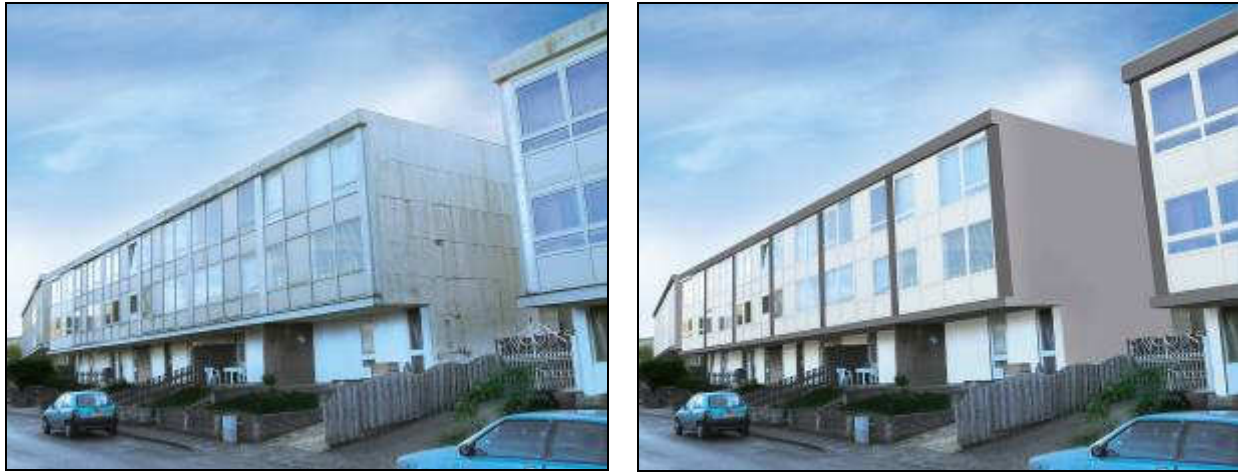
Figure: Impression of the dwellings before and after renovation
